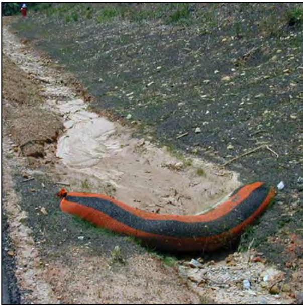
Sediment Tube used in a Ditch Setting
