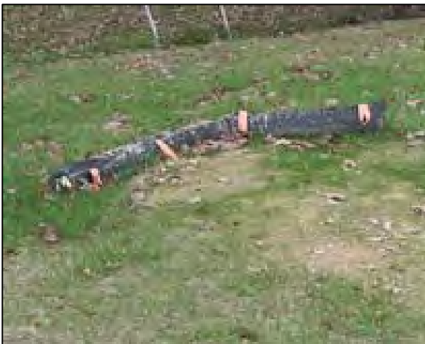
Sediment Tube used on Open Ground
