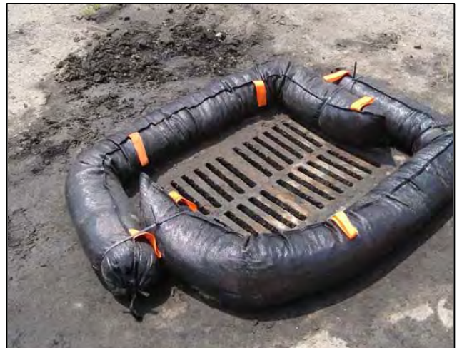
Sediment Tube used as Inlet Protection
