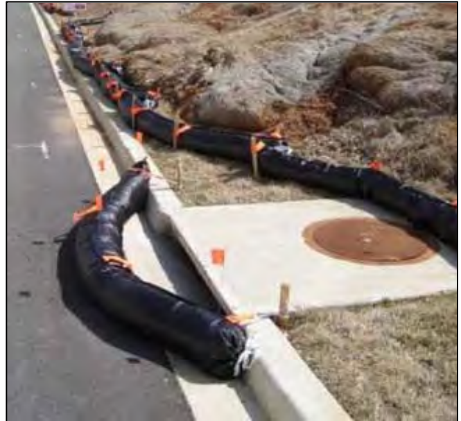
Sediment Tube used as Inlet Protection
