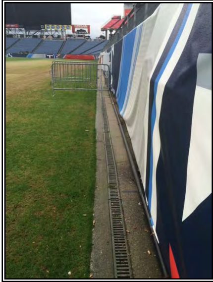
Trench Storm Drain around Field
