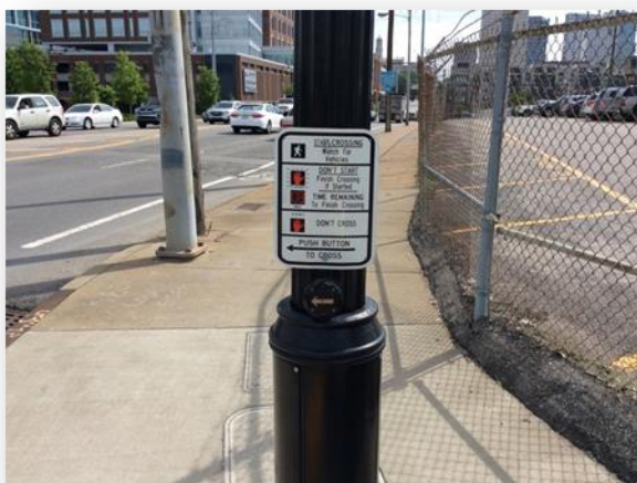
Push button with poor visual contrast, Charlotte Pike and George L Davis Boulevard
