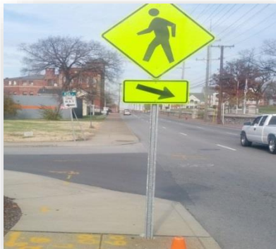
Sign is too low
