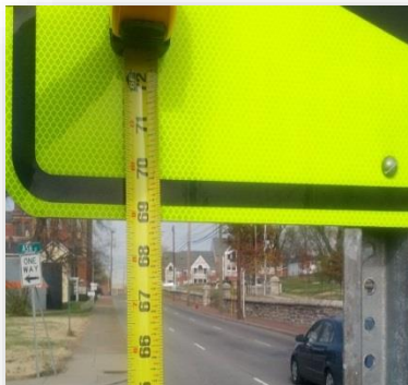
This sign barely qualifies, but it needs inventoried
