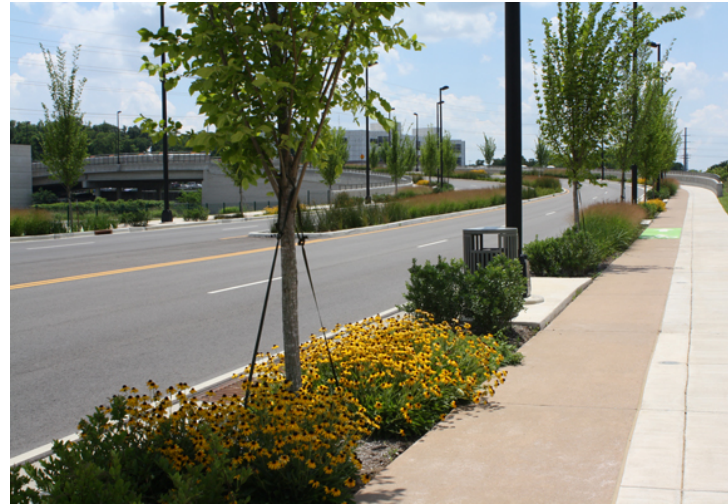
28th Ave Corridor: Complete street, bio-retention planters
