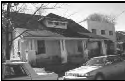
The residential buildings along the south side of Belcourt Avenue constitute a distinct and cohesive design character which contrasts with the north side of the street.
