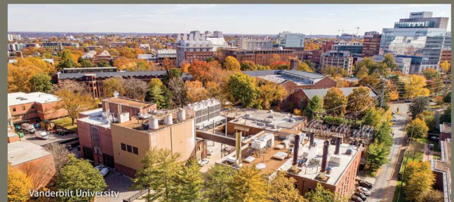
Vanderbilt University, winner of IDEA’s District Energy Space Award in 2020, opted to double down on district energy for its economy-of-scale advantages.
