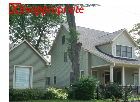
This house meets the lower eave height standard (B) but is too tall for the maximum height standard (A).
