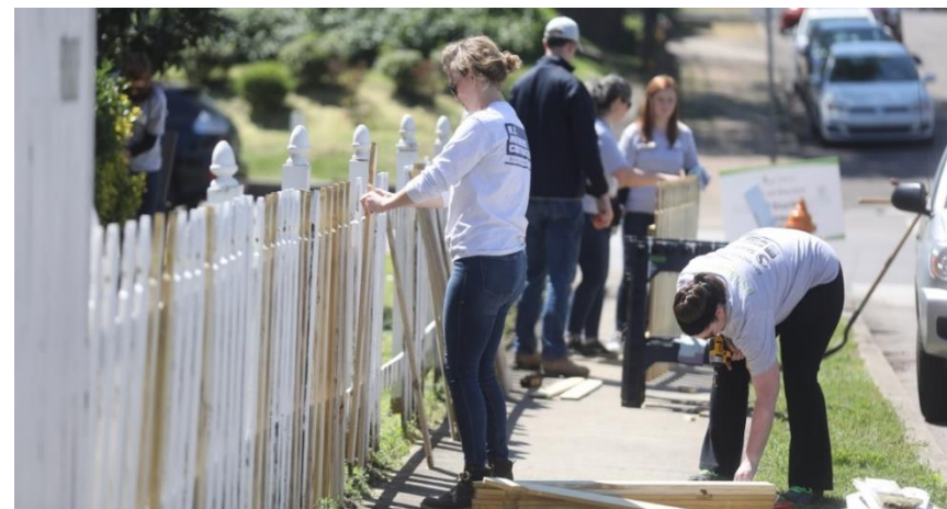
Rebuilding Together Nashville volunteers work on renovations for a local homeowner
