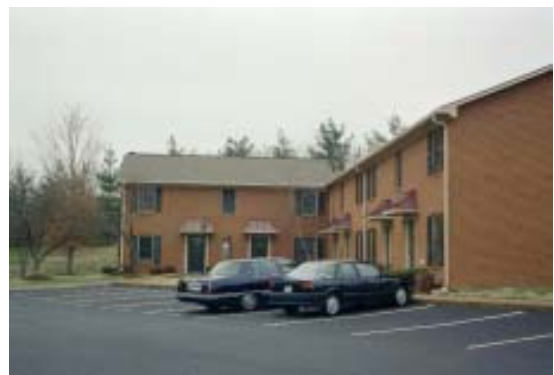
Multifamily near Bellevue Center
