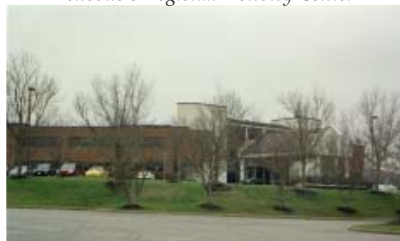
Offices such as this one adjacent to the Bellevue Center Mall are key components of Regional Activity Centers, as are residential uses
