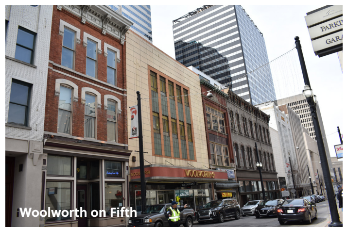
Kress Building - 5th Avenue
