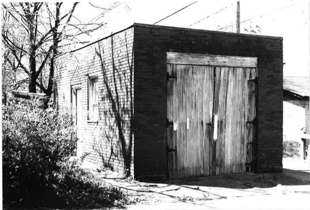
1115-17 Forrest: Single bay brick garage with a flat roof and vertical board double doors.
