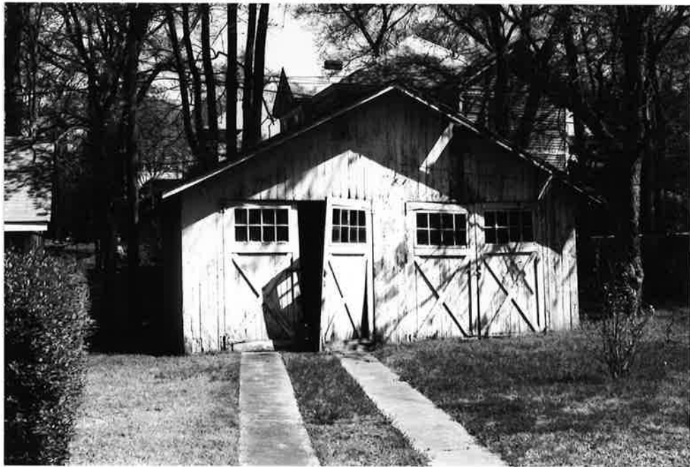
1403 Calvin: Gable roof frame two-bay garage with original glass and frame double doors.
