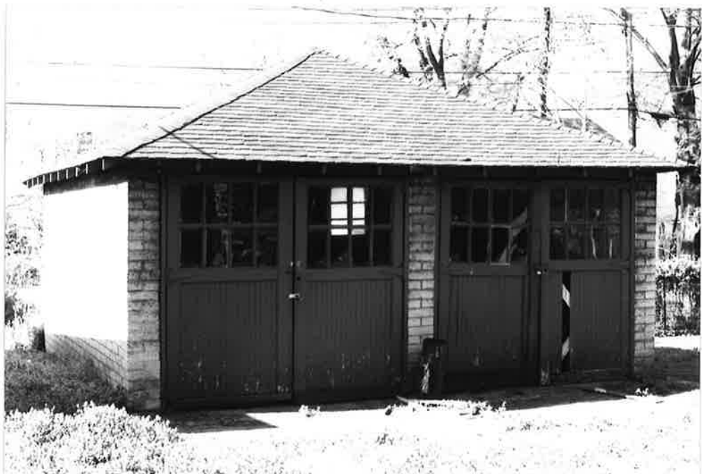
1204 Stratton: Brick garage with pyramidal roof and original glass and frame double doors.
