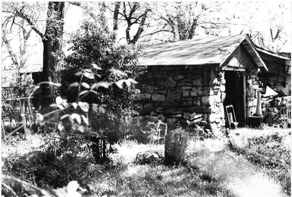
1403 Eastland: Stone veneer garage with a gable roof - is missing original doors.
