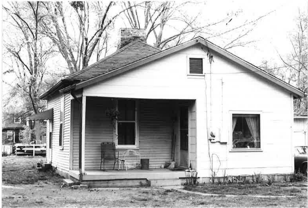
1501 Eastland: Remodeled servant's quarters at rear of main residence.
