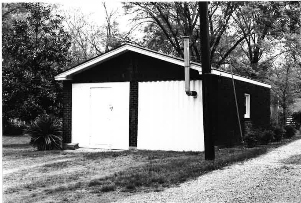
1411 Eastland: Brick garage with a gable roof and added modern doors and enclosures.
