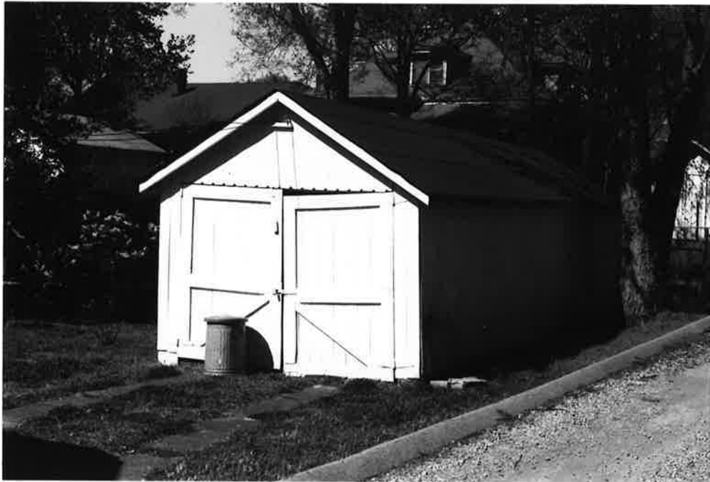
612 S. 17th St.: Gable roof frame garage with original frame, diagonal braced double doors.
