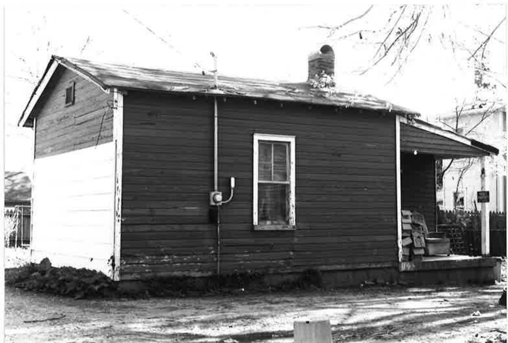
125 S. 11th St.: Original servant's quarters at rear of main residence.
