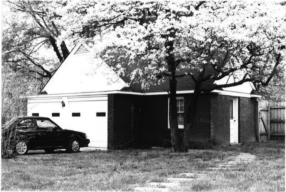
1415 Eastland: Brick garage with a gable roof and added modern overhead garage doors.
