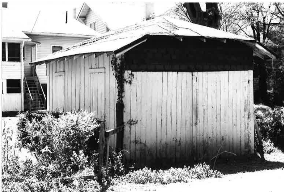
1109 Gartland: Frame garage with jerkinhead roof form variation and original vertical board double doors.
