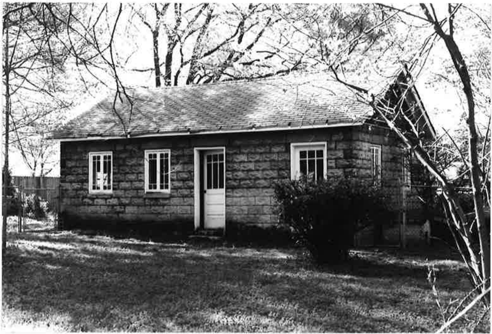
1500 Eastland: Hollow core concrete block garage with original doors and windows.
