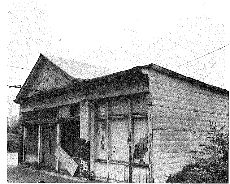
Fourth Avenue, North at Jackson Street
