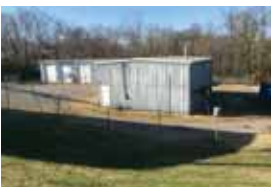
The existing metal buildings are to be relocated to an offsite location. The relocation of these buildings will be part of this contract.
