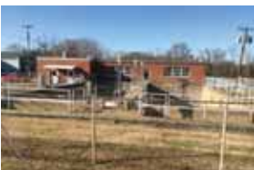
The existing Water Treatment Facility and sub-ground tanks are to be demolished and removed by Metro Public Works Department before the land is officially turned over to Metro Parks.
