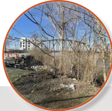
VIEW OF RAIL BRIDGE FROM TOP OF EMBANKMENT
