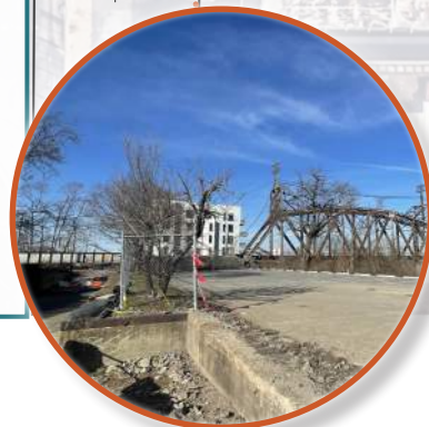
EXISTING CONCRETE WALL
