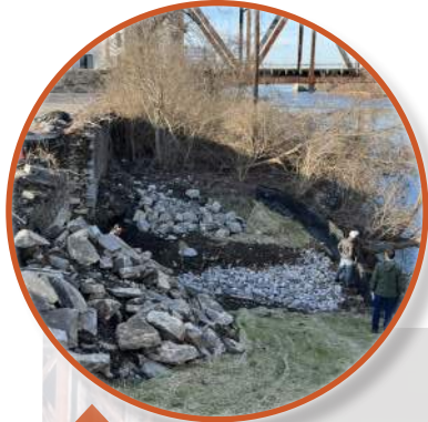
LOWER RIVER EDGE AND EXISTING STONE RETAINING WALL
