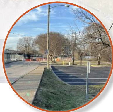
EXISTING GRADE CHANGE ALONG 1ST AVE. SIDEWALK
