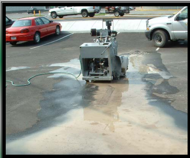
Pavement Cut Wet Saw Discharge
