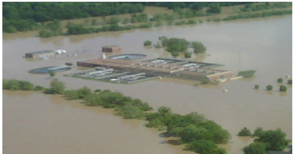
KR Harrington Water Treatment Plant under water
