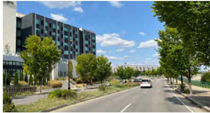
2 28th/31st Connector - Opened in Fall 2012, this street by One City has bike lanes next to the sidewalk, then they transition to on-street lanes. The street also has vegetated swales and street trees.
