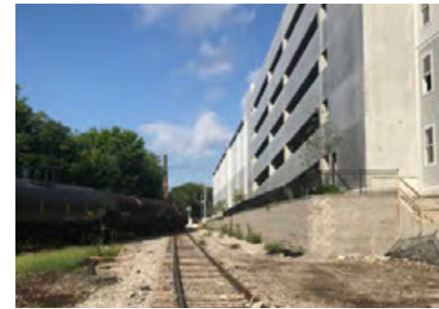
15 View looking north along the tracks behind new multifamily development.
