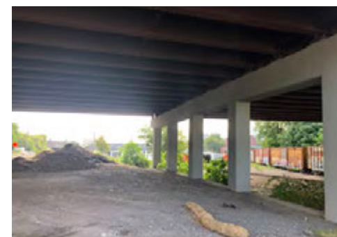
16 View looking east under the interstate 40 overpass.
