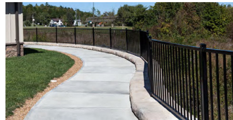
Note: safety railings may be needed in some locations.
