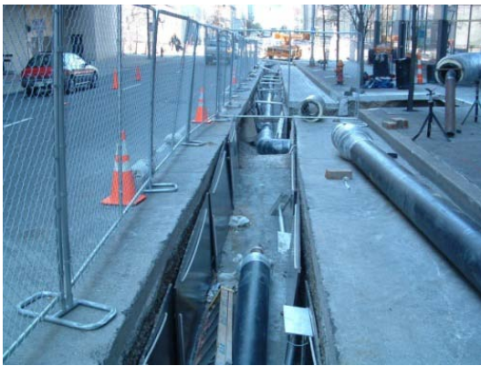
Manhole 5 to 9 Condensate Line Replacement
