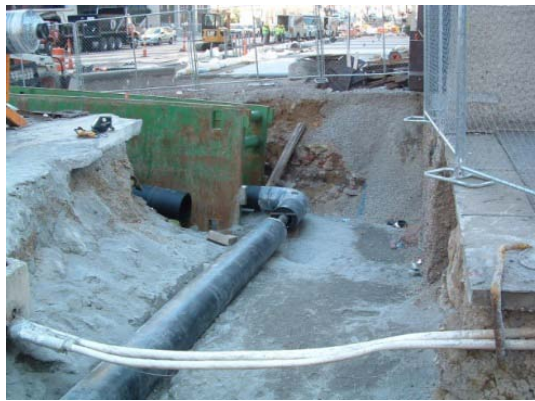
Manhole 5 to 9 Condensate Line Replacement
