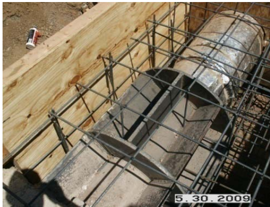
Manhole K Anchor Repair
