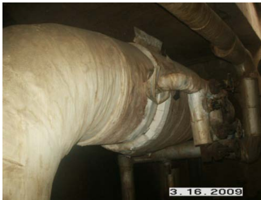
Manhole K before Modifications
