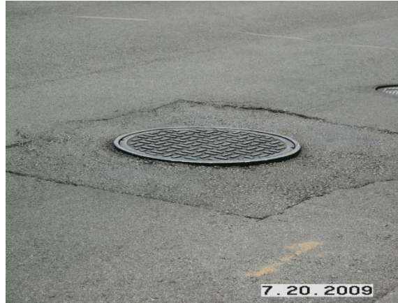
Manhole 13 Manhole Ring Replacement
