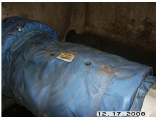
Manhole 6 Insulation
