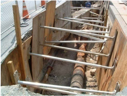
Manhole 6 to 23 Condensate Line Replacement
