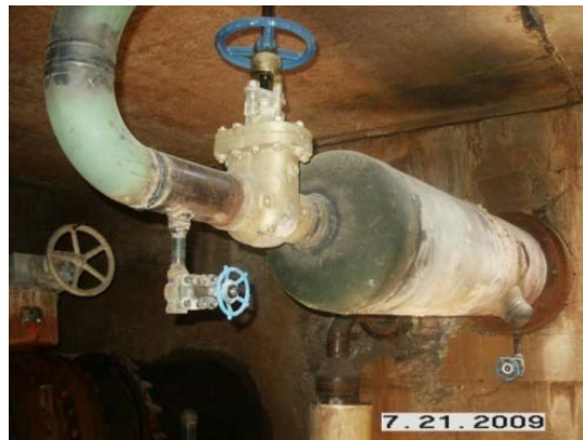
Manhole K after Modifications
