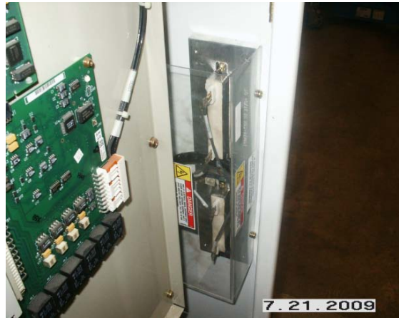
Chilled Water VFD Resistor Kit
