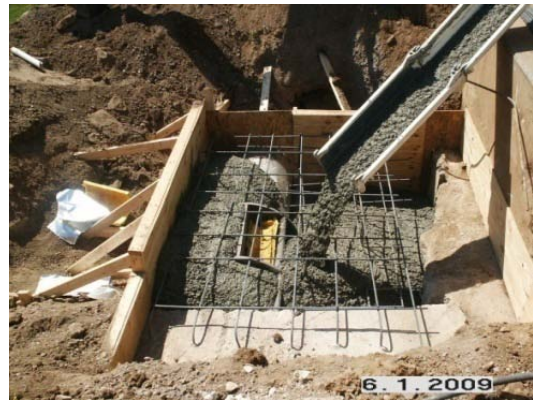
Manhole K Anchor Repair
