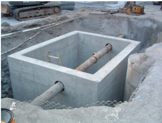
Manhole C - New Concrete Base and Frame
