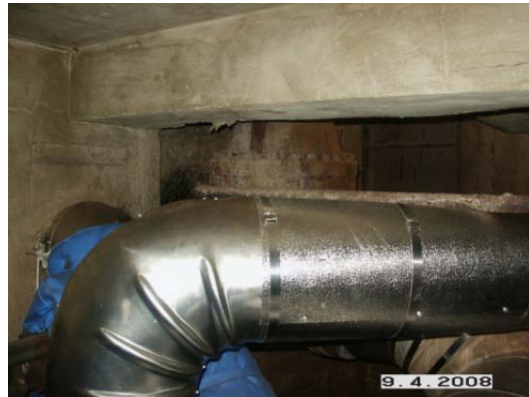
Manhole 10 Insulation
