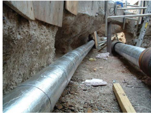
Manhole 6 to 23 Condensate Line Replacement
