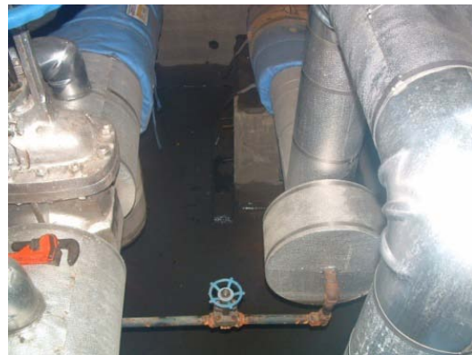
Manhole C - New Insulation
