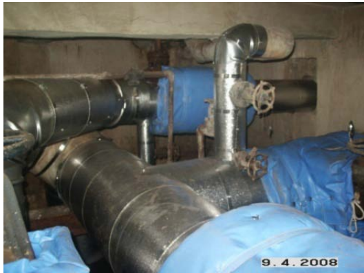
Manhole 10 Insulation
