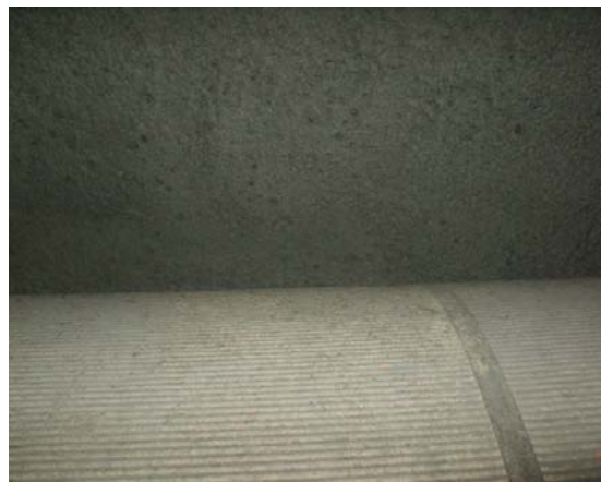
EDS Tunnel Structural Repairs-Broadway
