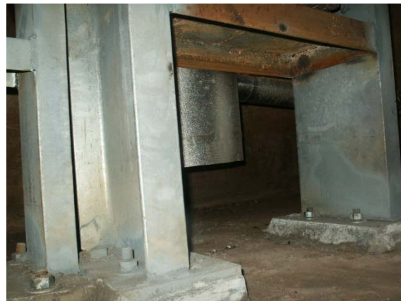
Manhole 1 Structural Steel Repairs
