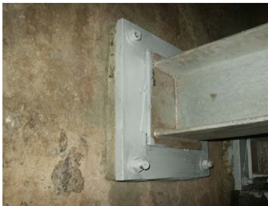
MH 13 Structural Supports
