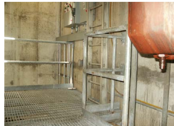
Platform Extension in Manhole 18
