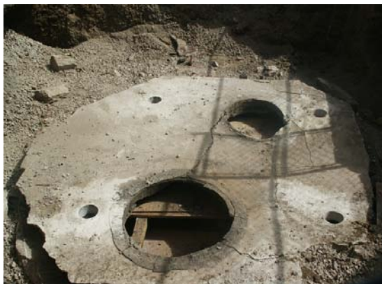
Manhole 12 lid before repairs
