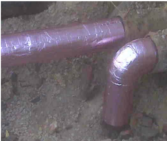
CJC Condensate Service Line Repair
