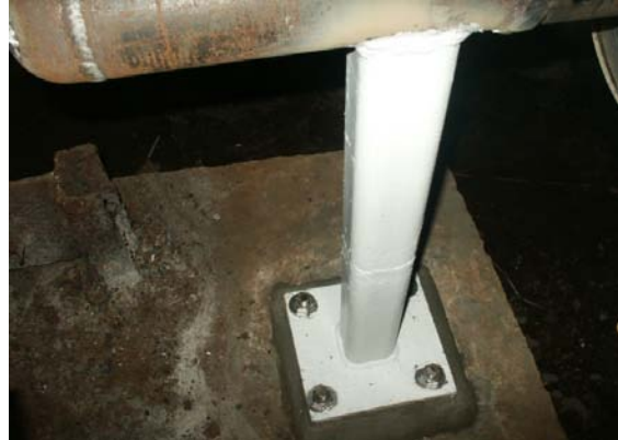
Manhole 4 Structural Repairs
