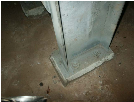
Manhole 1 Structural Steel Repairs
