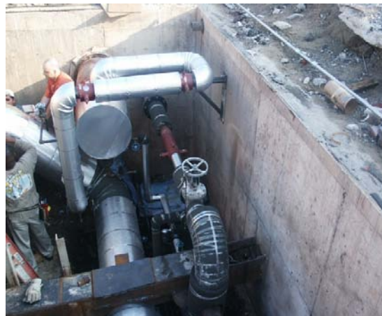
Manhole L Flood Damage Repairs
