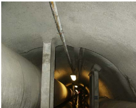
EDS Tunnel Structural Repairs-Broadway
