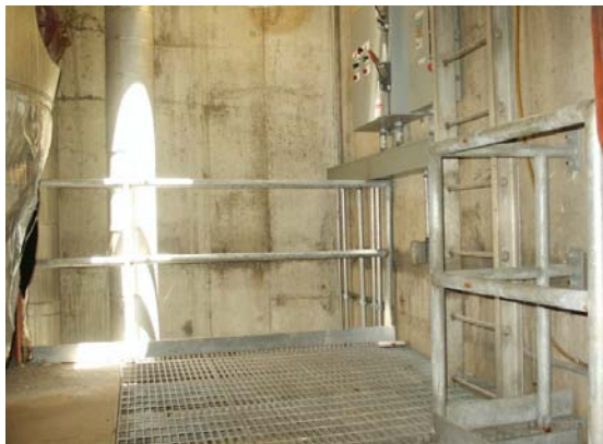
Manhole 18 Platform Extension
