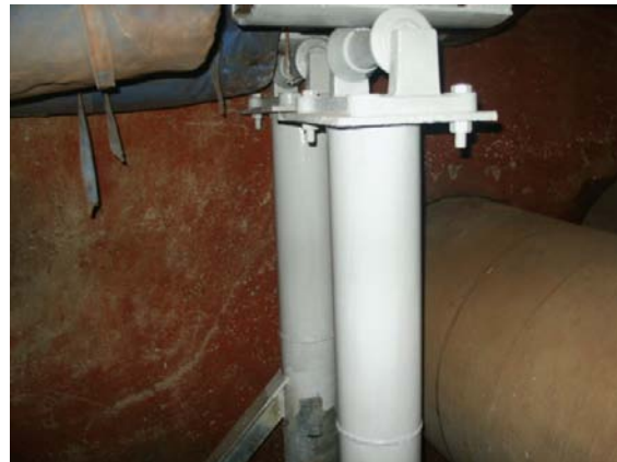
MH 13 Structural Supports
