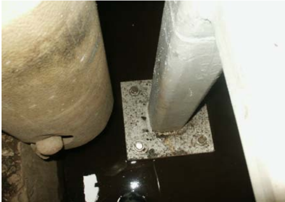
Manhole 3 Structural Repairs
