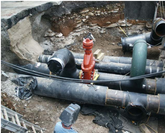
MCCC Chilled Water Piping
