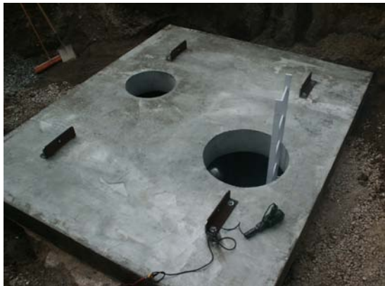
Manhole 12 lid after repairs
