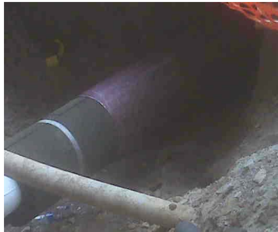
CJC Condensate Service Line Repair
