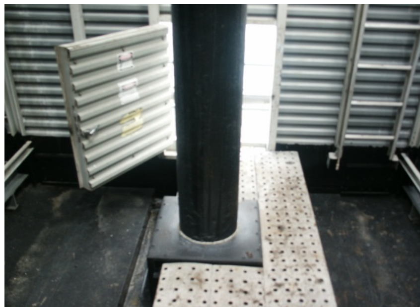
Re-coated the basins and riser pipes in Cooling Towers 10, 11, 15 and 18
