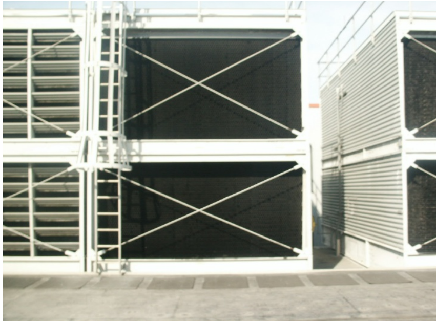
Installed new fill in Cooling Towers 10, 11, 15 and 18
