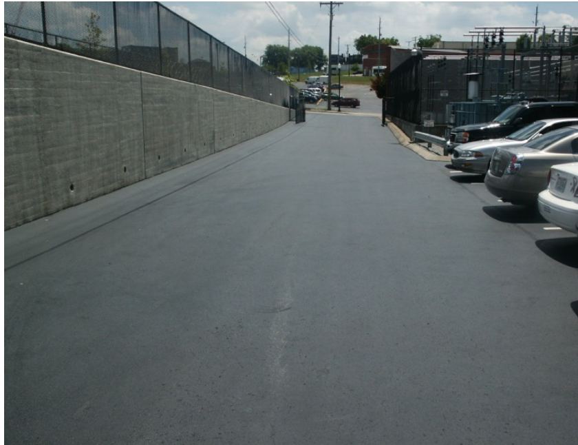
Sealed and Striped Parking Lot
