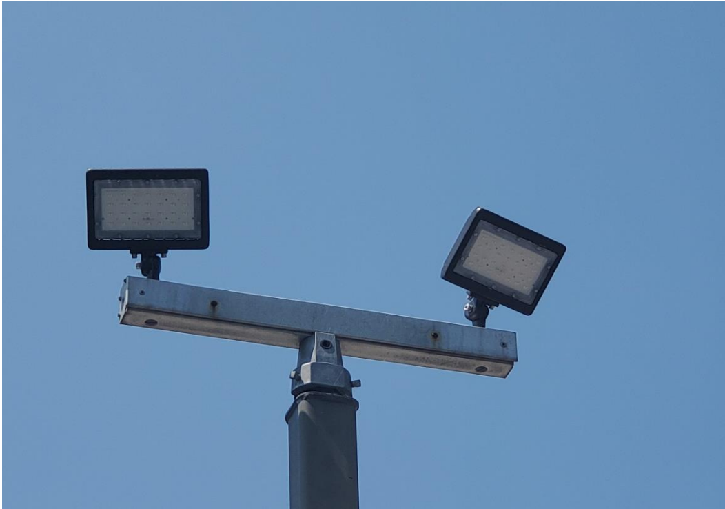
Switchyard Lighting Upgrade
