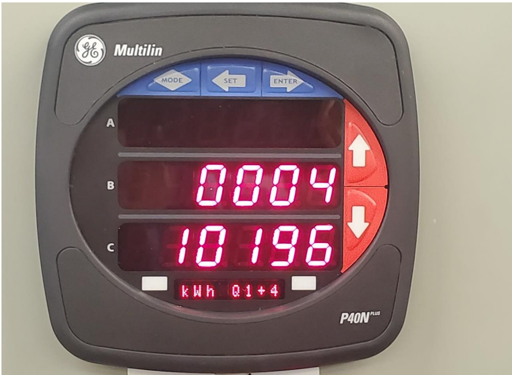
5B Switchgear Meter Upgrade
