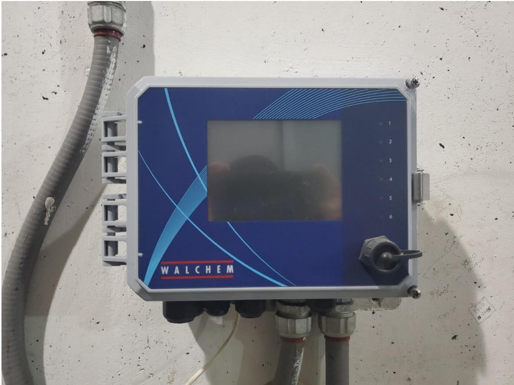
# 3 Boiler Conductivity Controller Upgraded (new panel)
