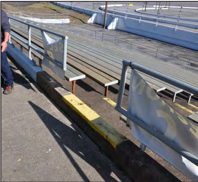
Upstand at the top of the bleacher steps
