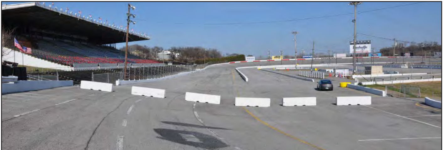
The pedestrian crossing over the speedway is quite steep on the outer edge
