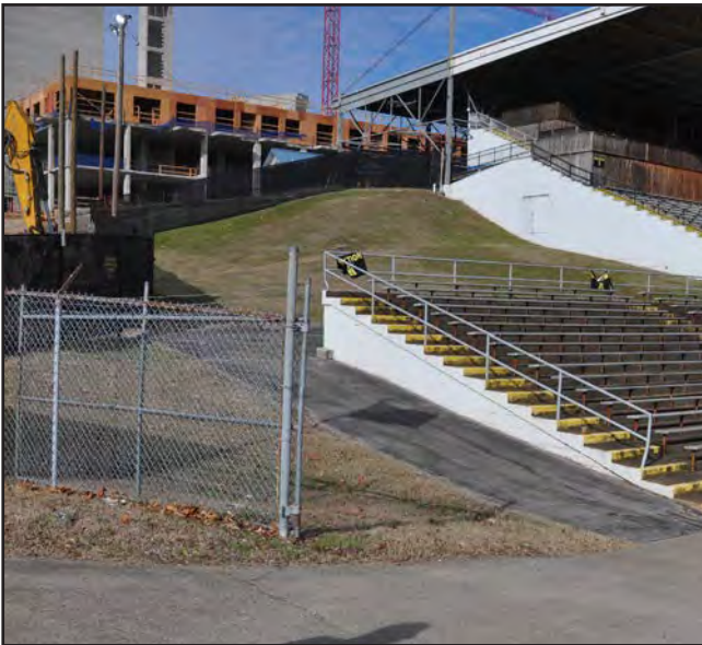
The grandstands sit on a steeply sloping site
