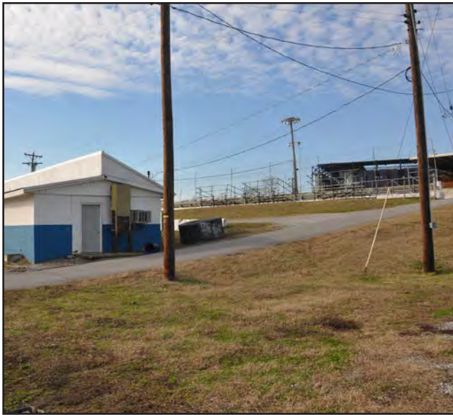
Steep slope leading to the mini bleachers on the infield
