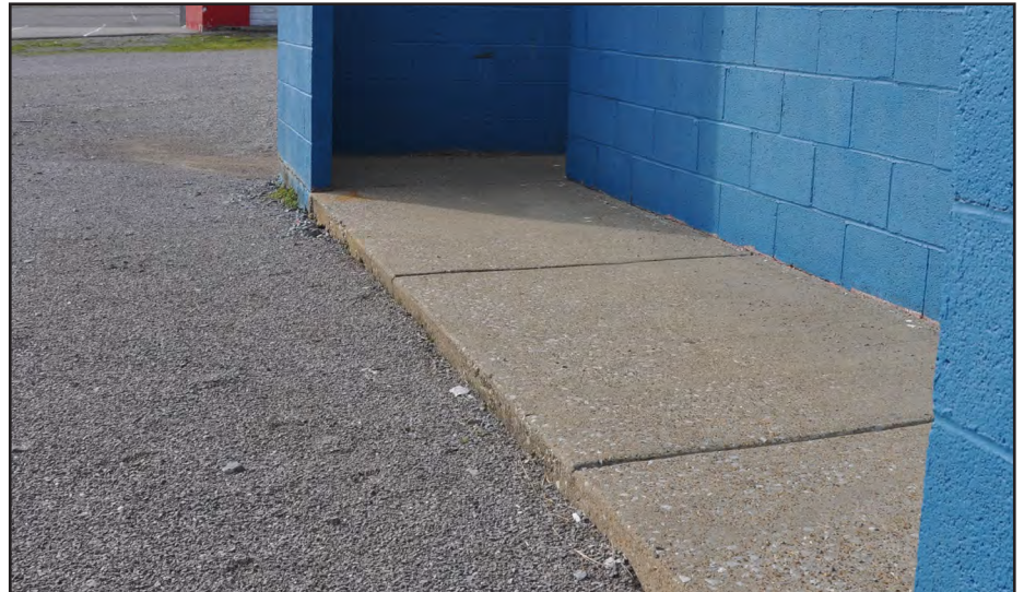
Small step up to infield restrooms
