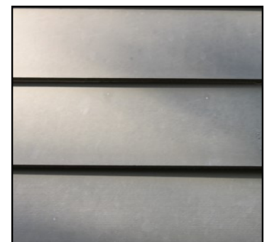
Fiber cement siding is an appropriate cladding for new construction but not when it has a faux (embossed) wood grain, as seen above. Below is an example of a smooth fiber cement siding that looks more like historic wood siding.
