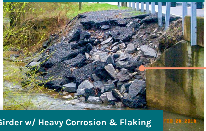
NE Embankment Failure
