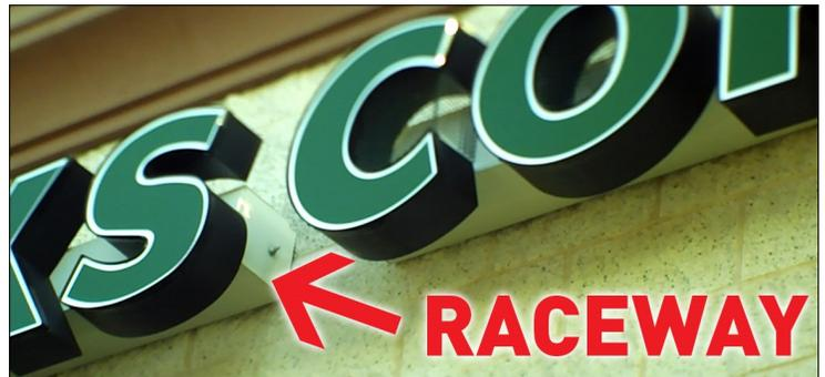
*Example of sign with exposed raceway.*
