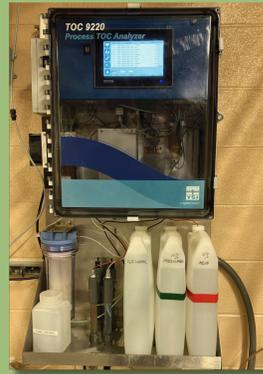
In 2023, Metro Water Services installed new on-line Total Organic Carbon (TOC) analyzers (YSI 9220) at both the Omohundro and K.R. Harrington Water Treatment Plants for continuous monitoring of raw and finished water.
