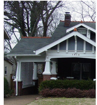
A porte-cochere is a covered entrance wide enough for a vehicle to pass through, typically opening into a courtyard. They are usually attached to the side of a building, one-story in height, and no more than 10'-12' wide.
