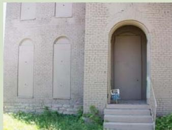
Any board placed on a vacant building shall be painted a color that is consistent with the color of the structure using exterior grade paint.
