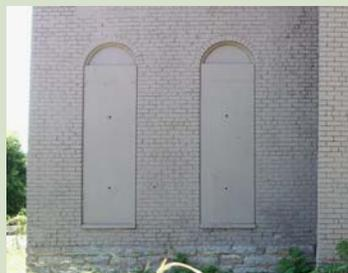
Any board placed on a vacant building shall be cut to fit into any windows, doors or other openings on such vacant building.
