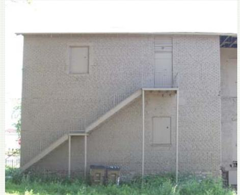
An example of a second story door opening that would require boarding because of access via the stairway from the ground level.
