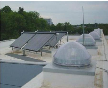
Roof top solar hot water heating panels are used to provide the facility with hot water, using the thermal energy of the sun.
