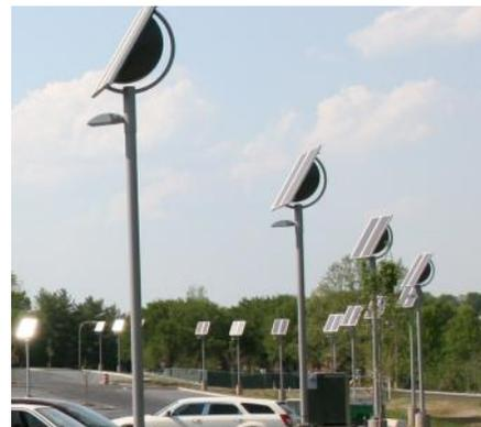
Solar powered, exterior lighting system designed to reduce the facilities carbon footprint by using free solar energy to light the exterior spaces of the facility.
