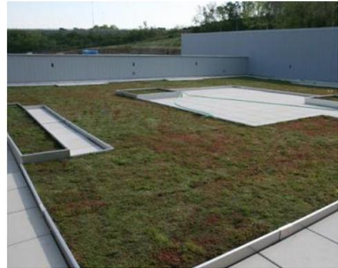
Detail of the "Green Roof" that features a vegetated area with heat absorbing plants, shrubs and small trees that will cool the air and provide insulating benefits and aesthetic appeal.
