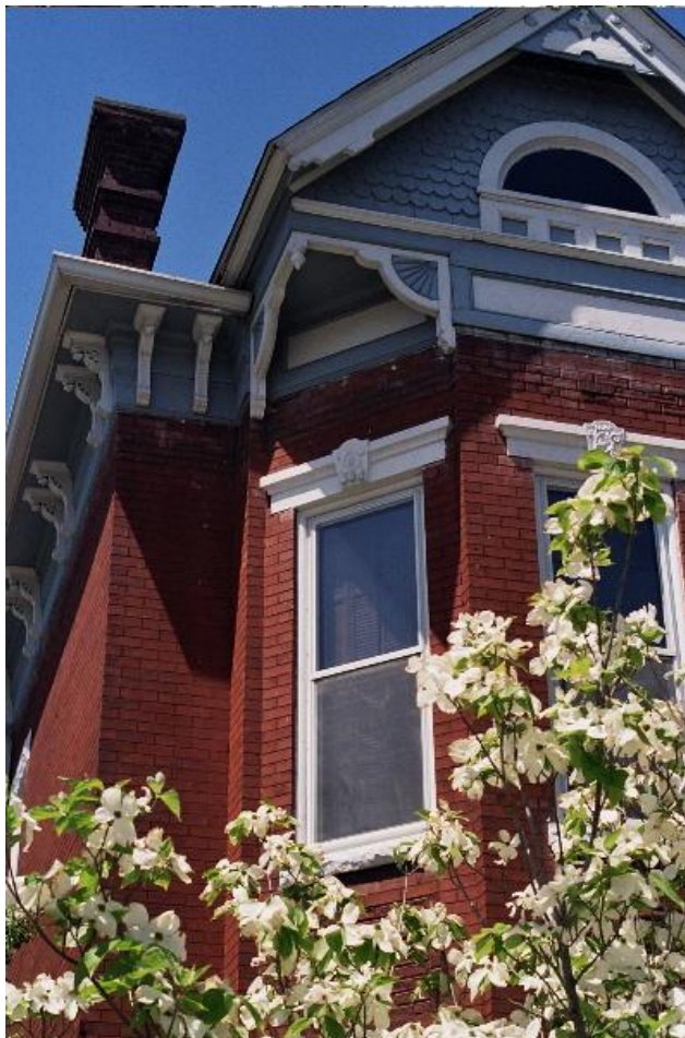
Storm windows can increase the energy efficiency of an older building and allow for the retention of the historic window
