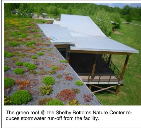
The green roof @ the Shelby Bottoms Nature Center reduces stormwater run-off from the facility.
