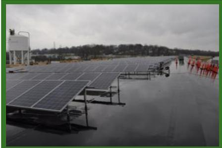
The rooftop array consists of 832 polycrystalline panels arranged in 32 parallel rows. The array is capable of generating enough energy to power approximately 50 average sized homes.
