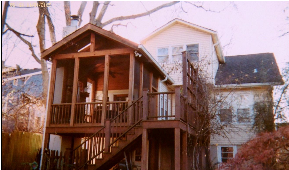
3620 Westbrook Avenue, rear.
