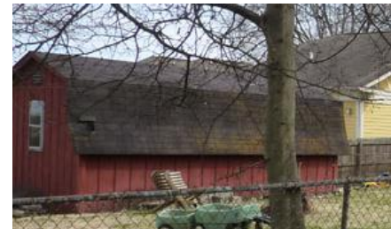
Figure 2. The outbuilding to be demolished.
