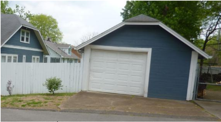
Figure 2. The 18 th Street façade of the existing outbuilding
