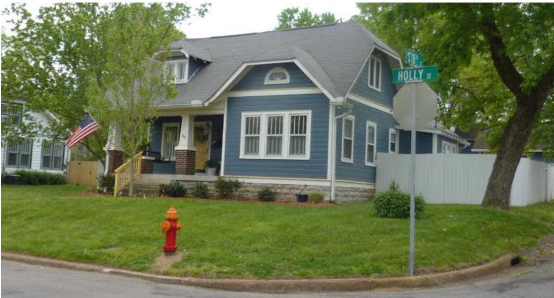
Figure 1. 1800 Holly Street primary structure.
