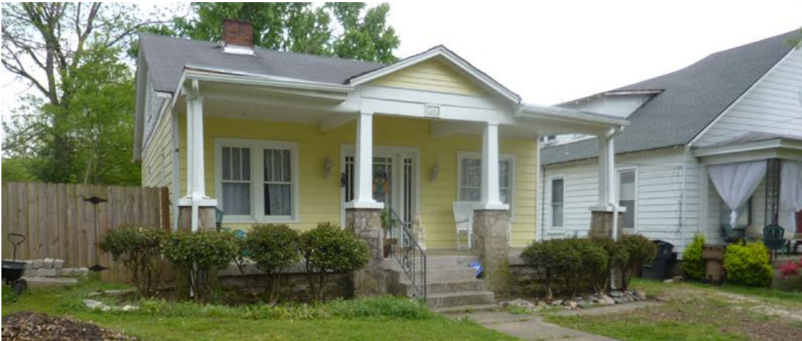
Figure 1. 1800 Holly Street primary structure.
