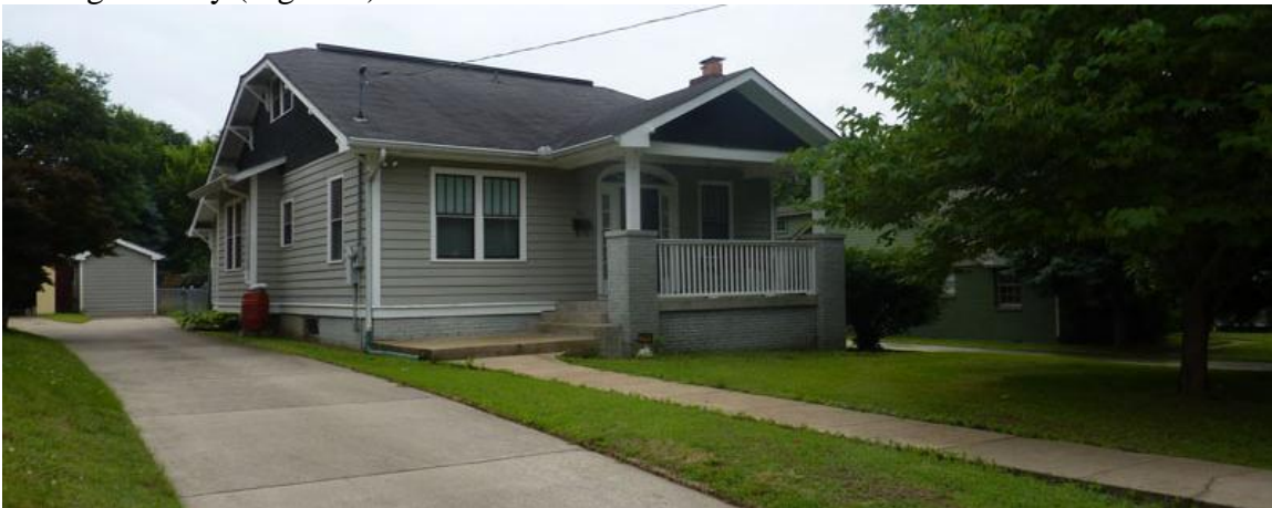
Figure 1. 415 North 15 th Street primary structure.
