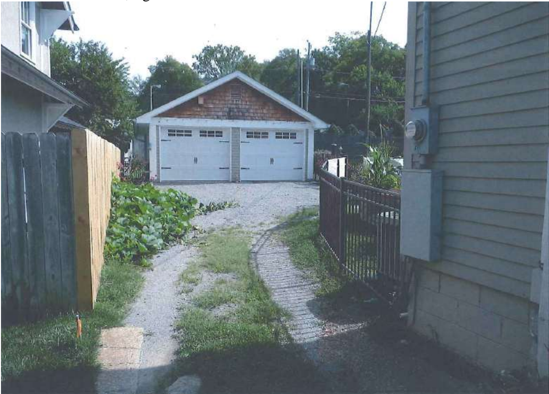
216 Fairfax Avenue, existing garage.
