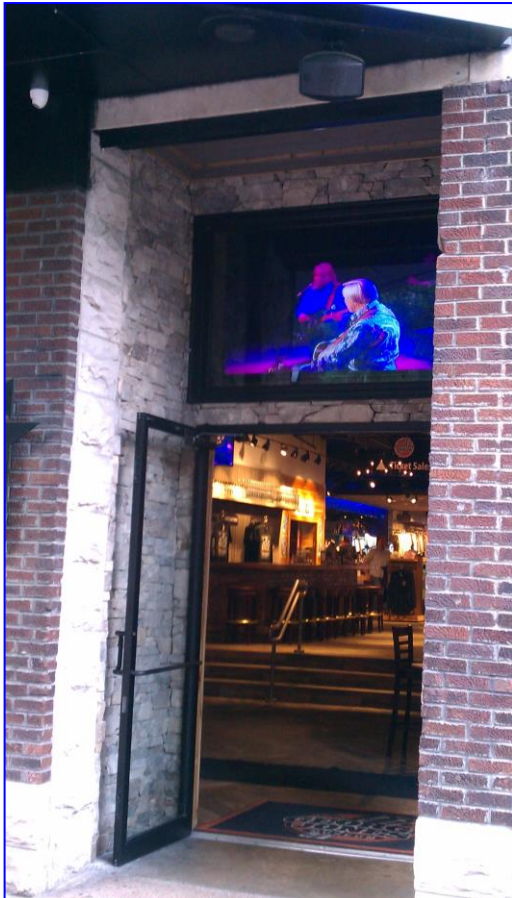
Figures 5 and 6: The left images shows the recessed walls of the primary entrance that has a veneer that was not approved and does not meet the design guidelines. The right image shows the secondary entrance on the Second Avenue side and the textured walls that were added.
