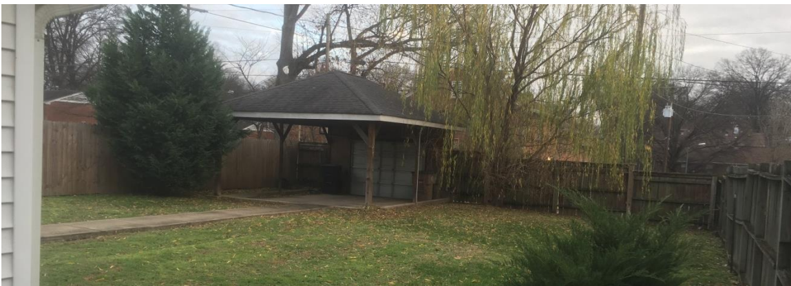
Figure 2 is the carport that is to be demolished.
