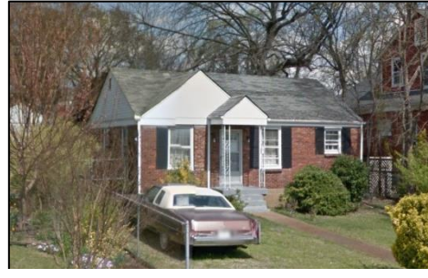
1404 Linden Avenue, existing building
