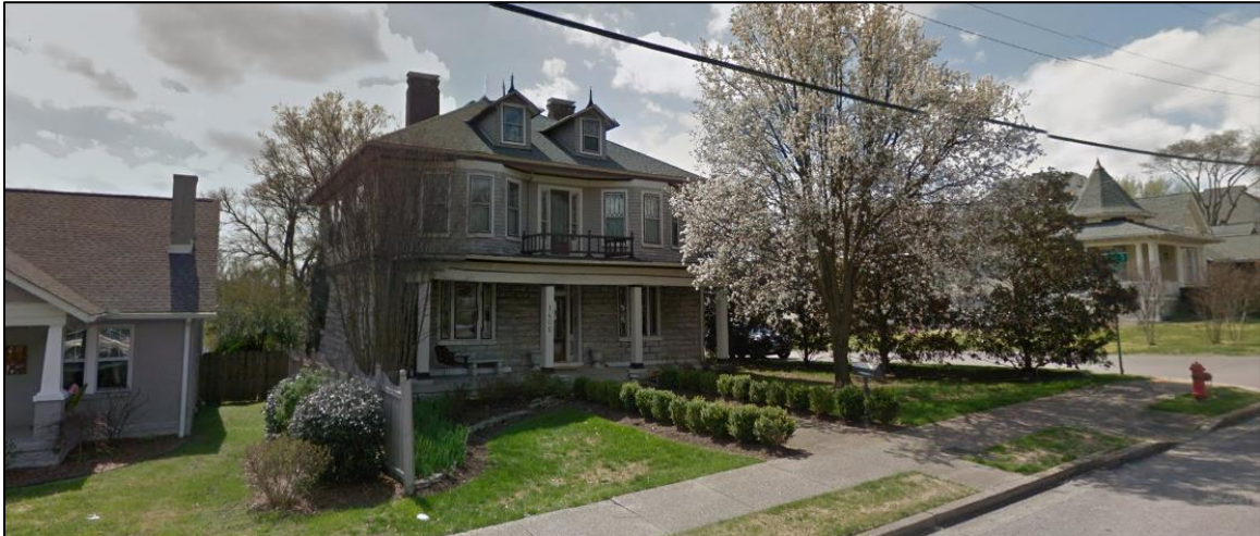
1405 Linden is two and one-half stories tall, but is on a fifty-nine foot (59') wide corner lot.
