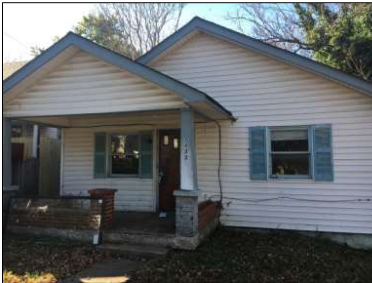
Figure 1. 1404 North 14th Street
