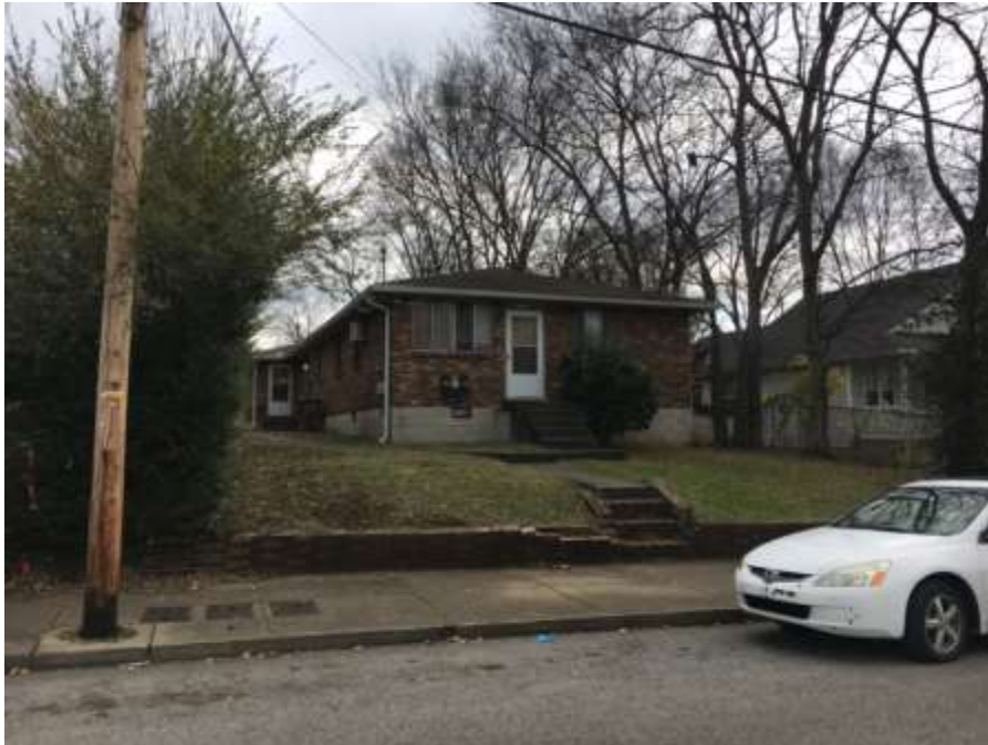
Figure 4. Non-contributing building at 1722 4th Ave N
