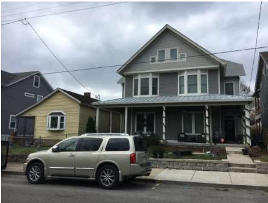
Figure 6. New construction at 1727 4th Avenue North
