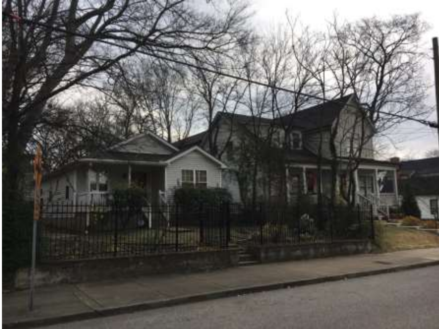
Figure 5. Nearest contributing building at 1716 4th Avenue North
