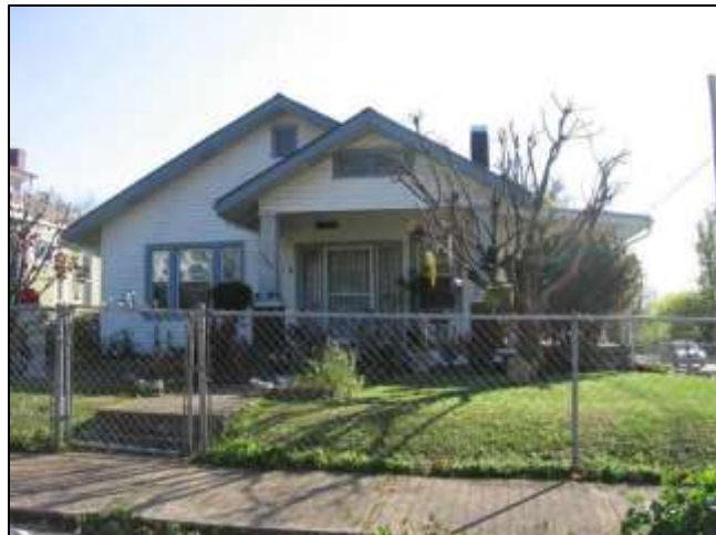
Figure 1. Contributing structure at 2000 Benjamin St
