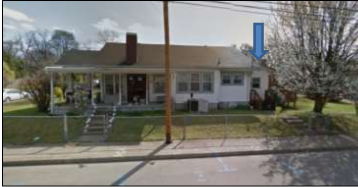
Figure 2. Existing rear addition at the right in this photo
