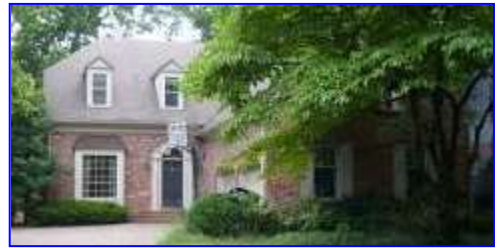
Figure 1: House as seen from the front in 2011, prior to alterations.
