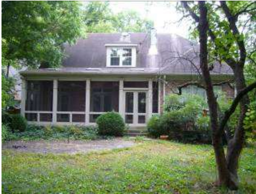
Rear of house taken from the back fence, prior to construction of the addition.
