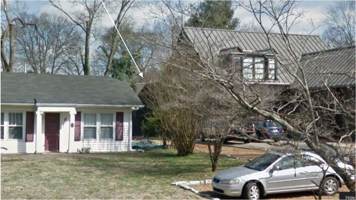
Rear addition prior to the installation of the green-wall.
