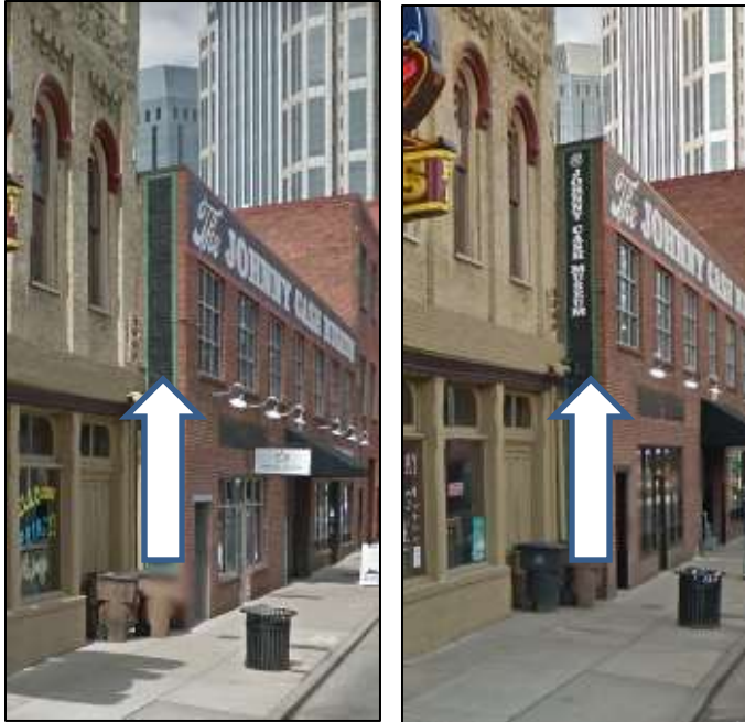
Figures 1 and 2: Left image is the building in April 2014 and the right is the building is March 2015.
