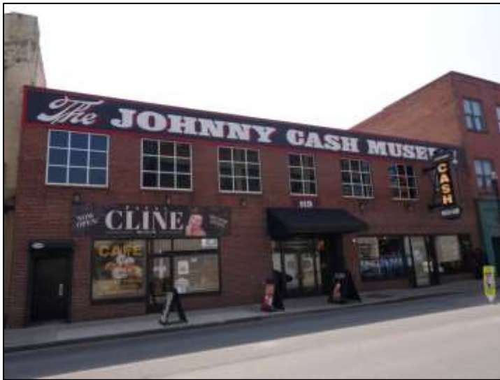
Figure 5. Existing signage at 119 3rd Avenue S showing that the reduction in painted signage was never accomplished although the projecting sign was installed.
