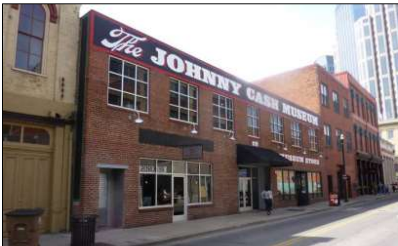
Figure 3: Conditions at the time of approval of the projecting sign. Approval of projecting sign was based on the painted sign located above the second level windows being reduced in square footage so that the two sign types together met the allotment.
