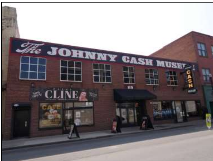
Figure 5. Existing signage at 119 3rd Avenue S showing that the reduction in painted signage was never accomplished although the projecting sign was installed.
