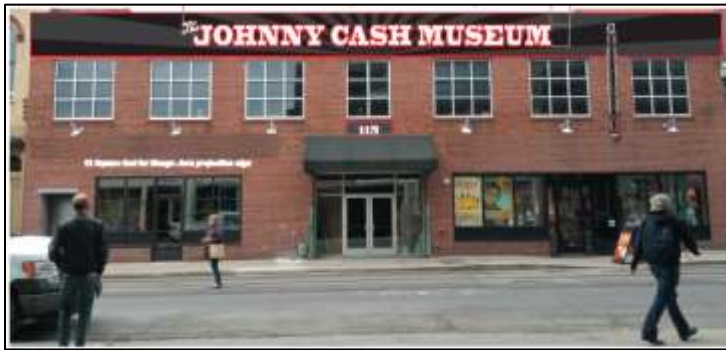
Figure 4. Per the permit issued in 2015, the painted sign was to be reduced to 105 sq ft, to match image shown above, allowing the building to meet its allocation of sign area
