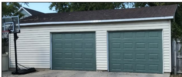
Figure 3: Existing garage to be demolished
