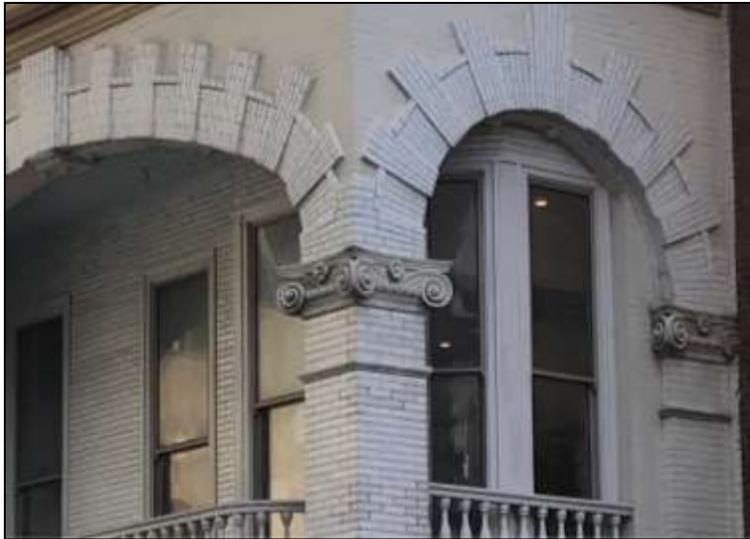
Figure 9. A detail of the glazed brick and terra cotta at the second level.
