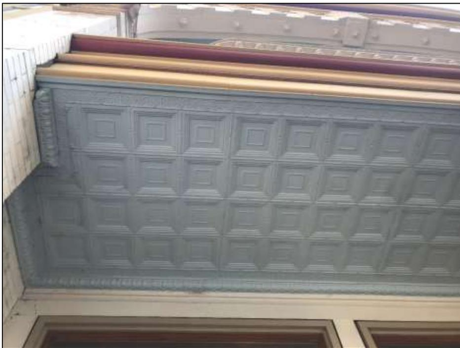
Figure 10. The coffered ceiling above the storefront.
