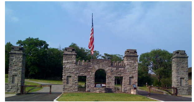
Entry Gates Constructed by the WPA
