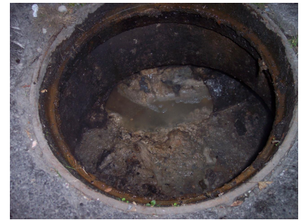
Sewer line blockage from grease.
